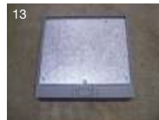
13 To convert the trap suitable for tile application, cut the tile according to the size of the trap.
