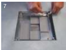
7 Adjust the leveling screws to the screeded or desired level. Secure both frame & trap simultaneously
