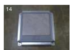
14 If tile is thicker than the recess, grinding is necessary. Remove the throw-away lid and install the frame & trap
